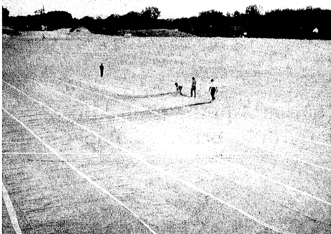
IN THE PIT: A plastic liner was laid in the bottom on the new burial cell at Chelsea's sanitary landfill last week. It looked something like a foot-
